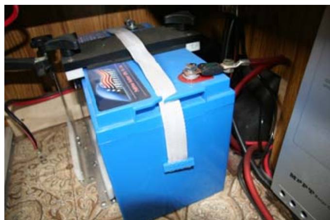
Battery securely mounted close to the controller.
